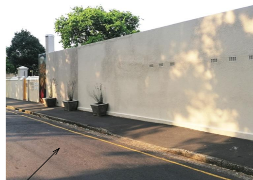
Street elevation with entrance at the end
