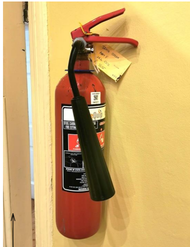
fire extinguishers are inadequate fire control & will damage the artworks
