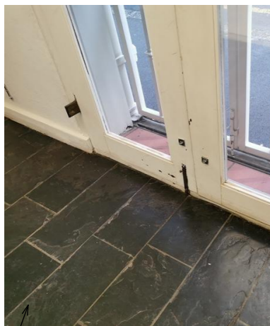
Slate tiling in previous entrance hall
