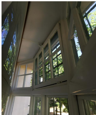
Bay window in Dudley's Room with UV blind
