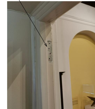
Internal door to Dudley's Room removed
