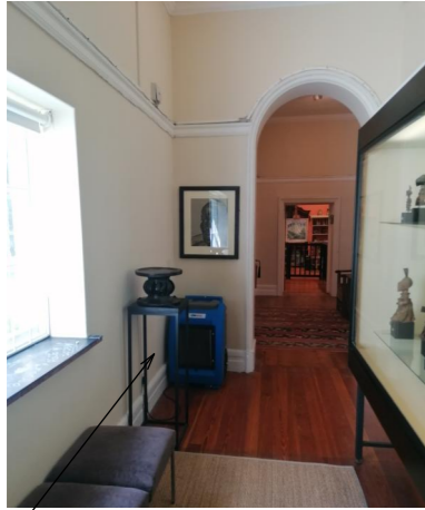
The dehumidifiers are an inadequate long term solution to environment control
